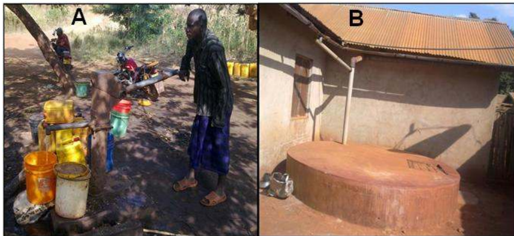
Plate 1. Bore hole (A) and rain water harvest (B) as sources of water in Kabuku Ndani ward
